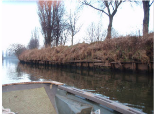
Downstream length: general view
